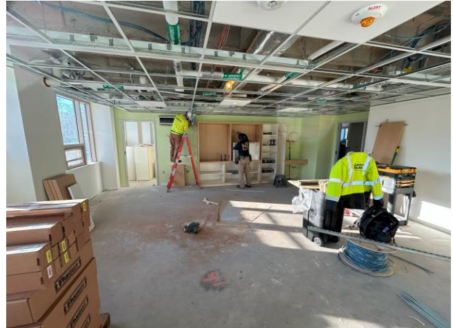
Ceiling grid and casework, floor 3
