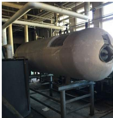
Original storage tank abandoned in place
