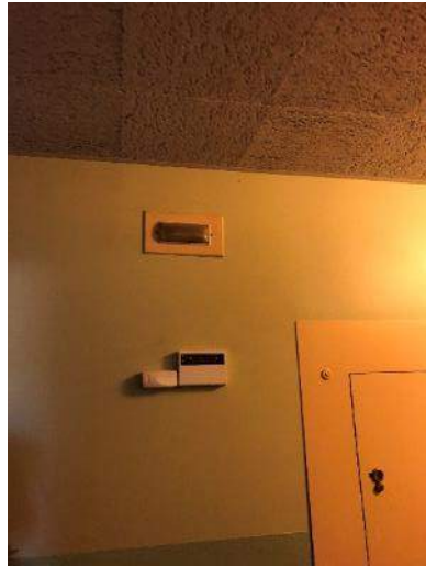
Normally Off Emergency Light Fixture
