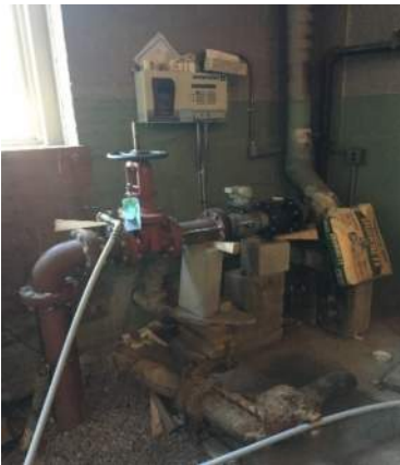
New backflow preventer with concrete block used as support.
