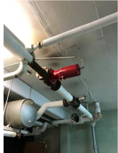
Convent Hot Water Circulator Pump
