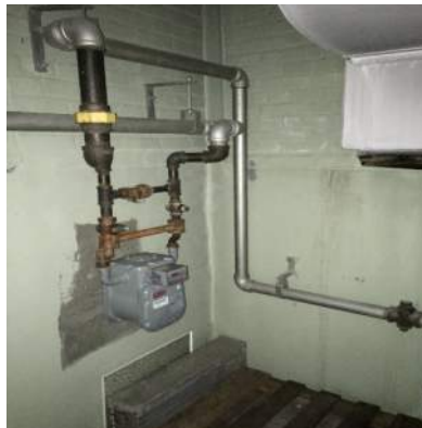
Gas meters in boiler room, below cafeteria Gas meter in the old convent area
