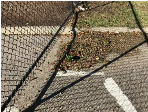
Photo 13: One of the observed catch basins on site located near the parking on the south side of the building, covered in leaves
