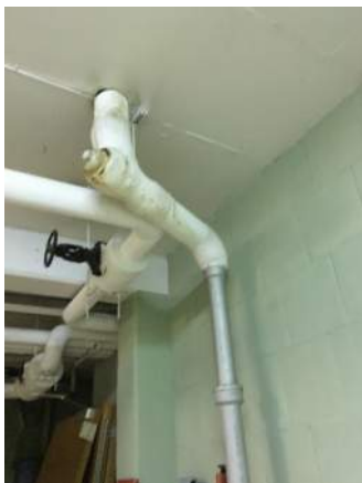
Waste pipe in boiler room
