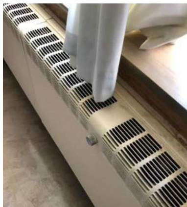
Hot water Fin tube Radiation
