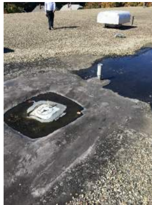
Roof drain with water puddles
