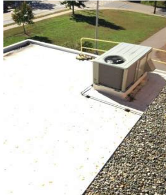
Gas feed to RTU's
