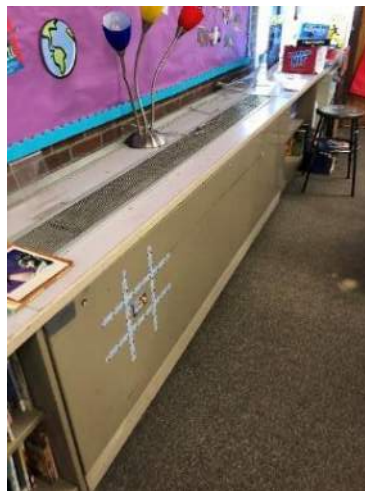
Hot Water Unit Ventilator
