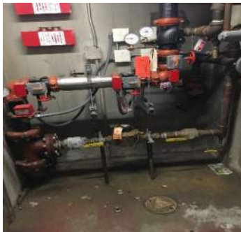
Water service entrance with backflow
