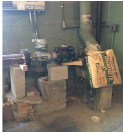
New backflow preventer with concrete block used as support.
