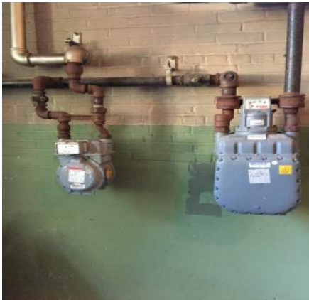
Gas meters in boiler room, below cafeteria Gas meter in the old convent area
