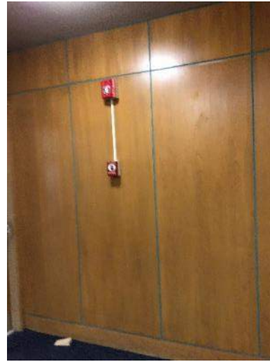
Fire Alarm Notification Appliance & Non-ADA compliant pull stations
