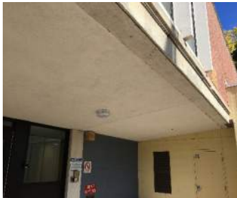
Exterior canopy with no sprinklers
