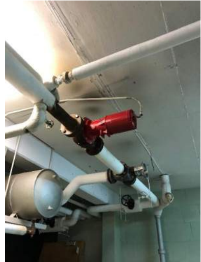
Convent Hot Water Circulator Pump
