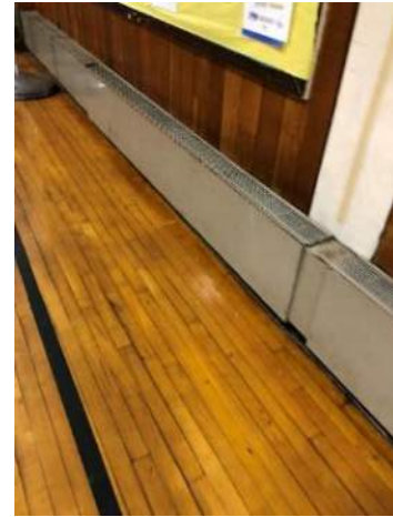
Gym Fintube Radiation Heating
