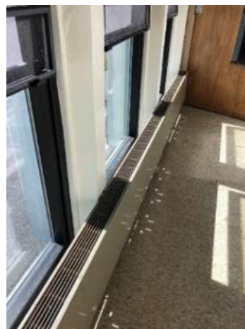
Corridor Fintube Heating
