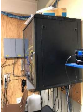
Tel/data wiring rack
