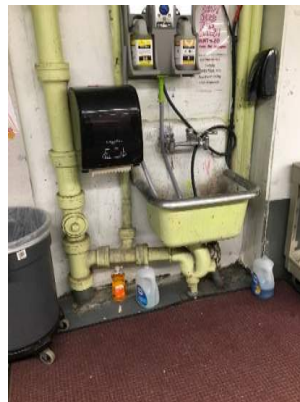
Waste pipe with mop sink connection
