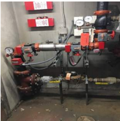
Domestic water service entrance with no backflow preventer
