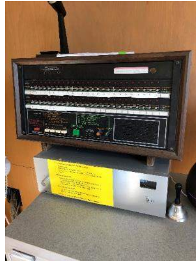
Intercom System Head End
