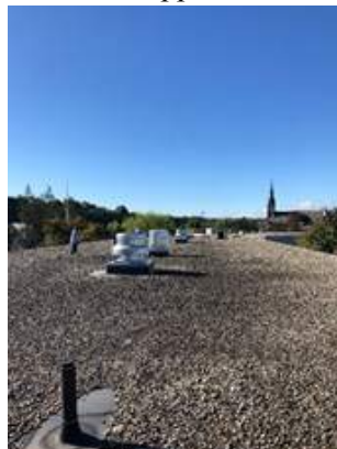
Roof Exhaust Fans
