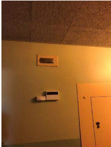
Normally Off Emergency Light Fixture
